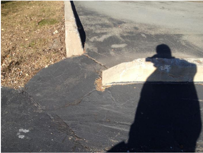
Curb cut drainage to adjoining creek, southwest corner of site.
