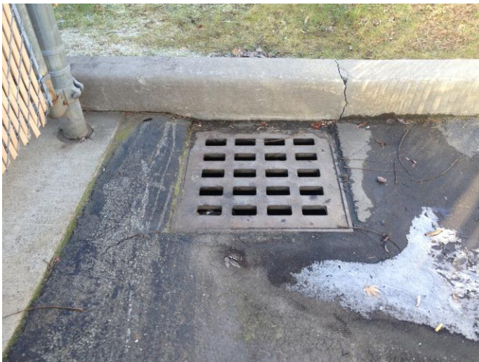
Storm drainage catch basin adjacent trash enclosure.
