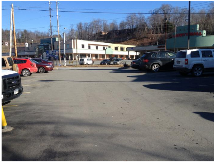
Composite view of subject structure from the northwest.
