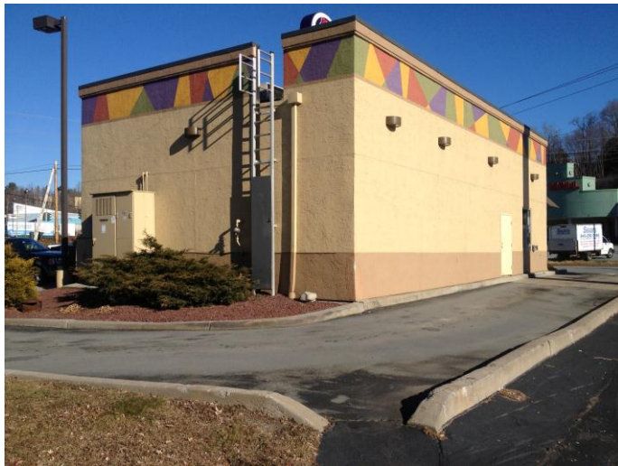
View of subject property from the southwest.
