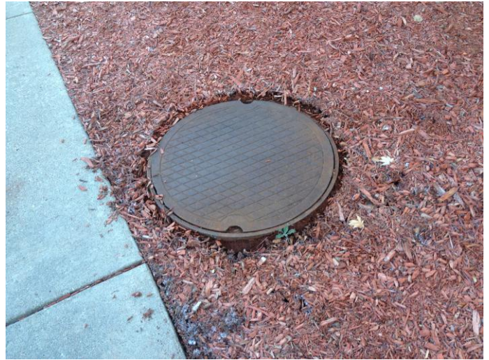
Underground grease trap north of onsite structure.
