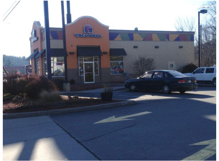
View of parking lot and structure from the northeast.
