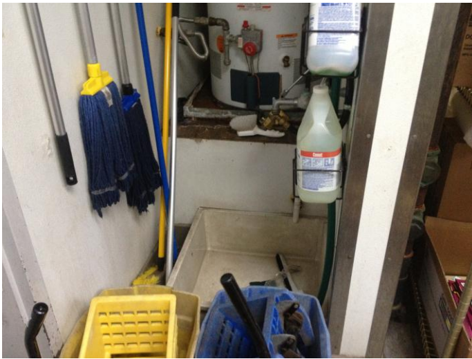
View of mop sink.
